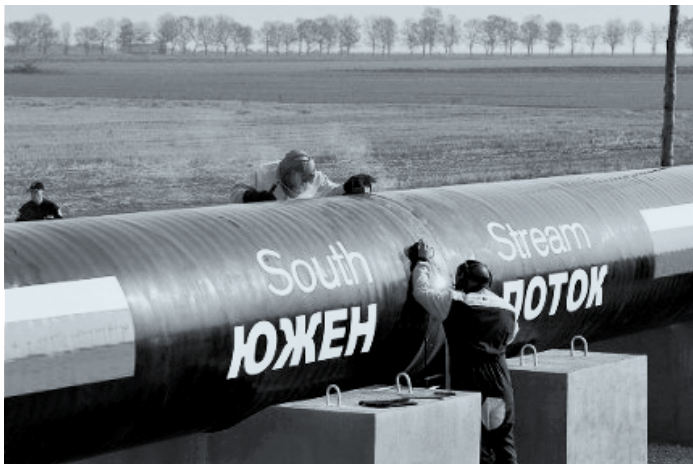
Bulgarian section of South Stream pipeline under construction
